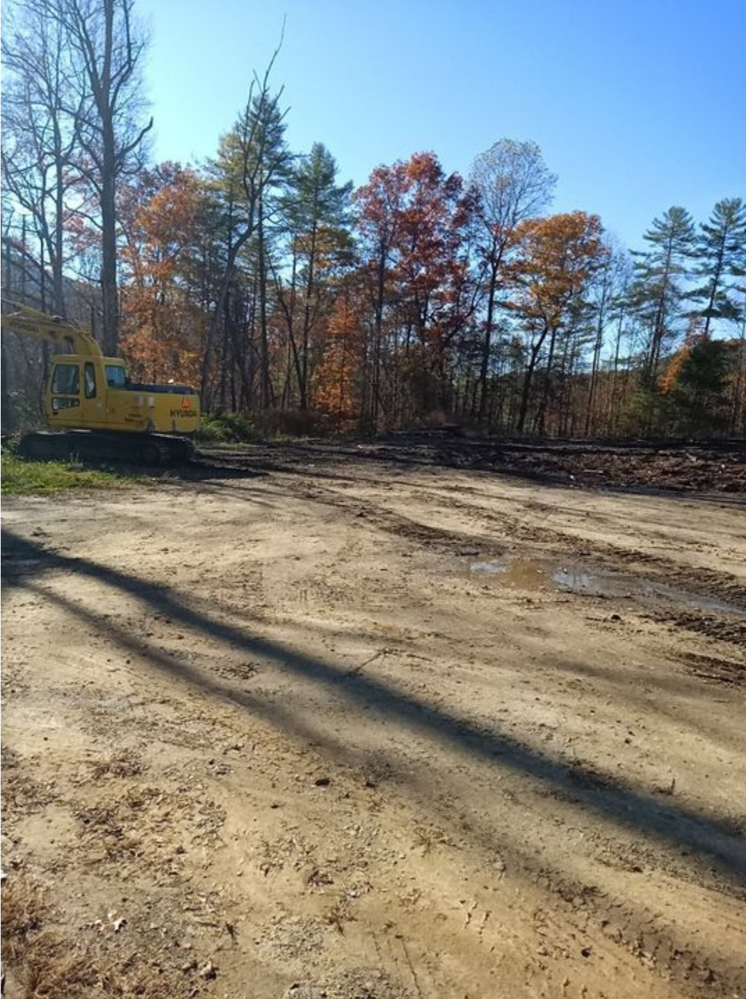
Image #4 Text: Clearing and grubbing.
